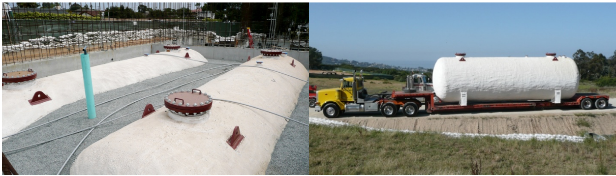
FIGURE 12. PRIMARY TES TANK INSTALLATION AT THE JCVI BUILDING, SAN DIEGO, CA
