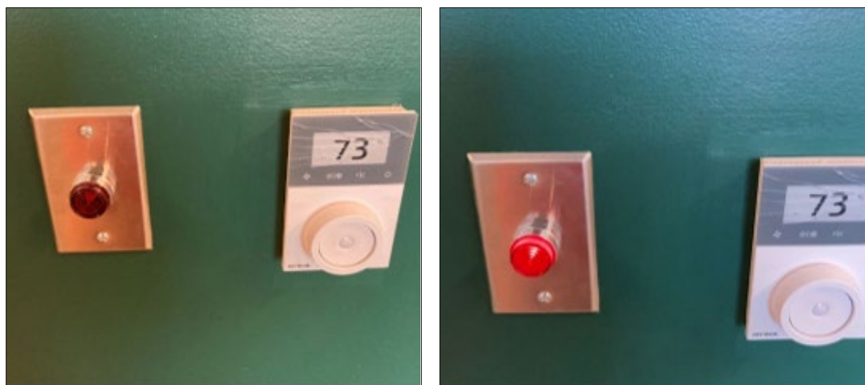
FIGURE 34: RTU FDD TRIGGERED (LEFT), ALARM AT ZONE LEVEL ADJACENT T-STAT (RIGHT)
