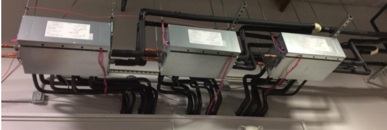
FIGURE 3: VRF SYSTEM HEAT RECOVERY REFRIGERATION BRANCH UNITS
