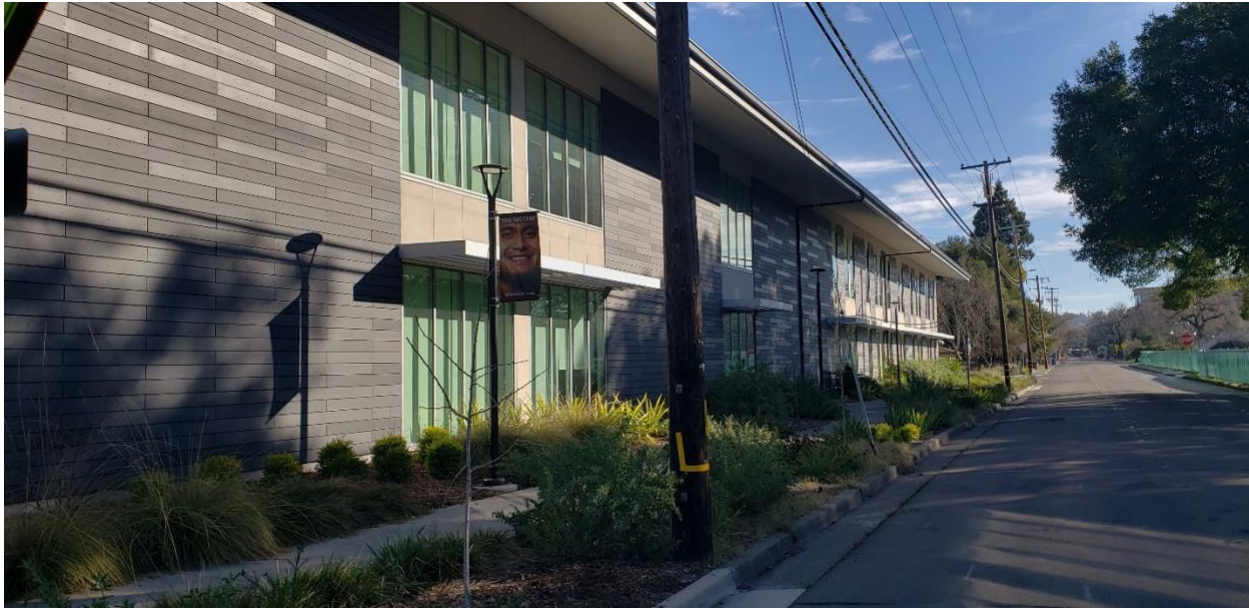
FIGURE 1: BUILDING A EXTERIOR
