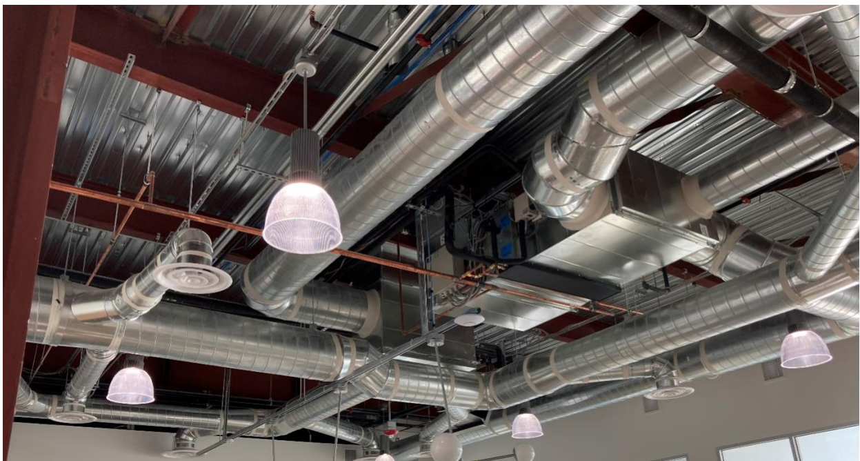
FIGURE 5: VRF DUCTED FAN COIL
