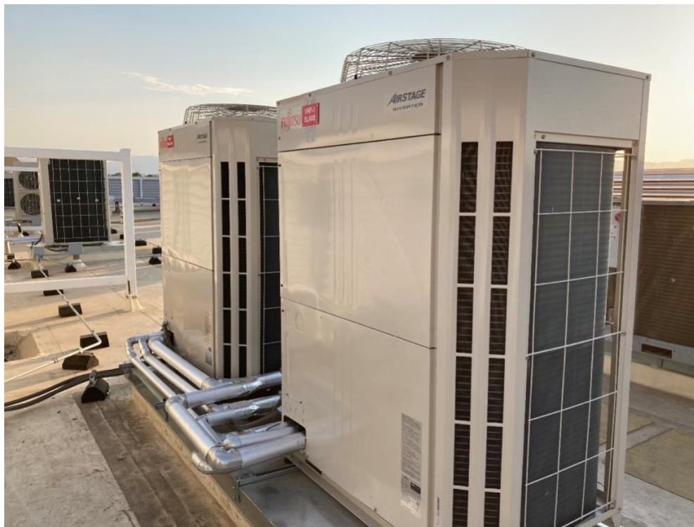
FIGURE 3: VRF MULTI-ZONE OUTDOOR HEAT PUMPS
