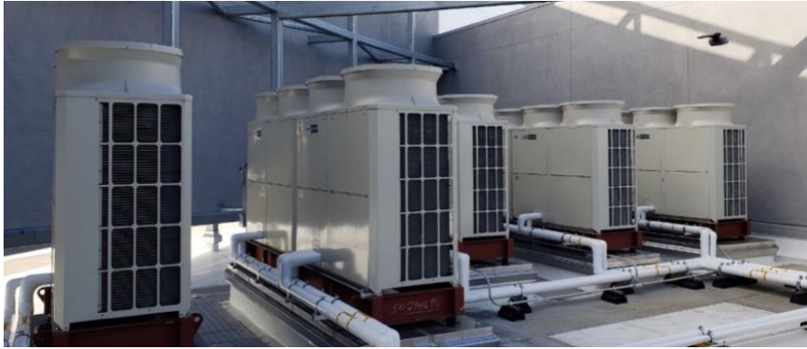
FIGURE 1: VRF AIR SOURCE HEAT PUMPS
