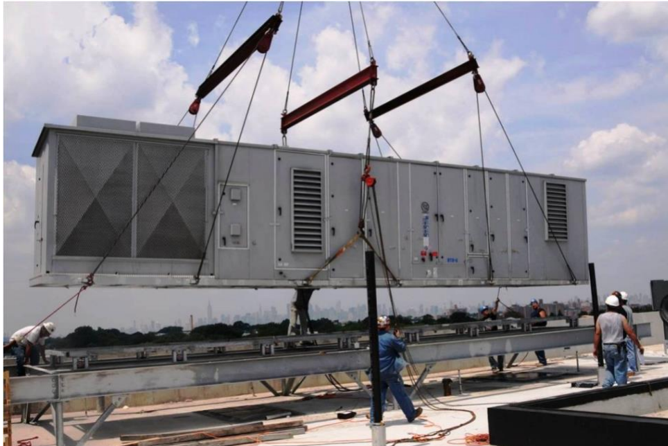
FIGURE 2: PACKAGED AIR-TO-AIR HEAT PUMP
