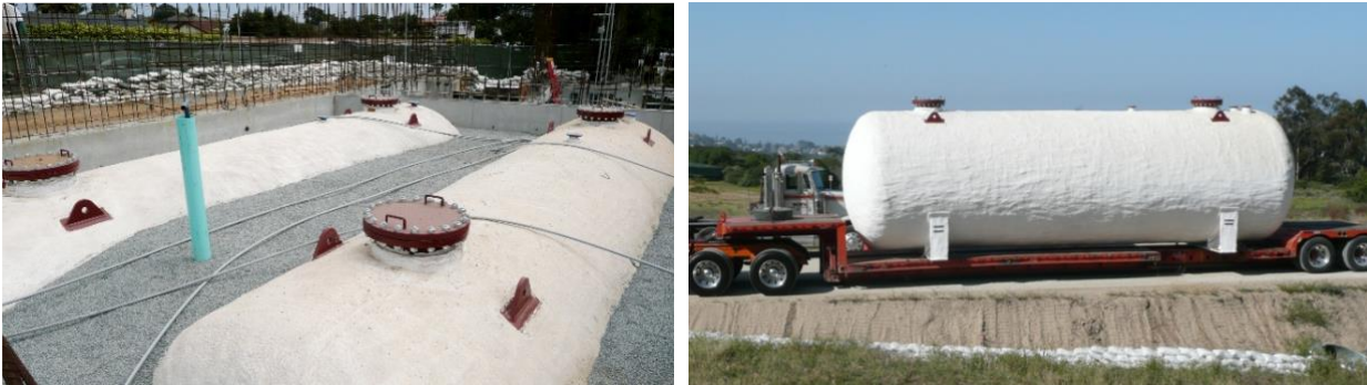
FIGURE 11: THERMAL STORAGE TANKS IN A COMMERCIAL BUILDING FOR HEATING AND COOLING
